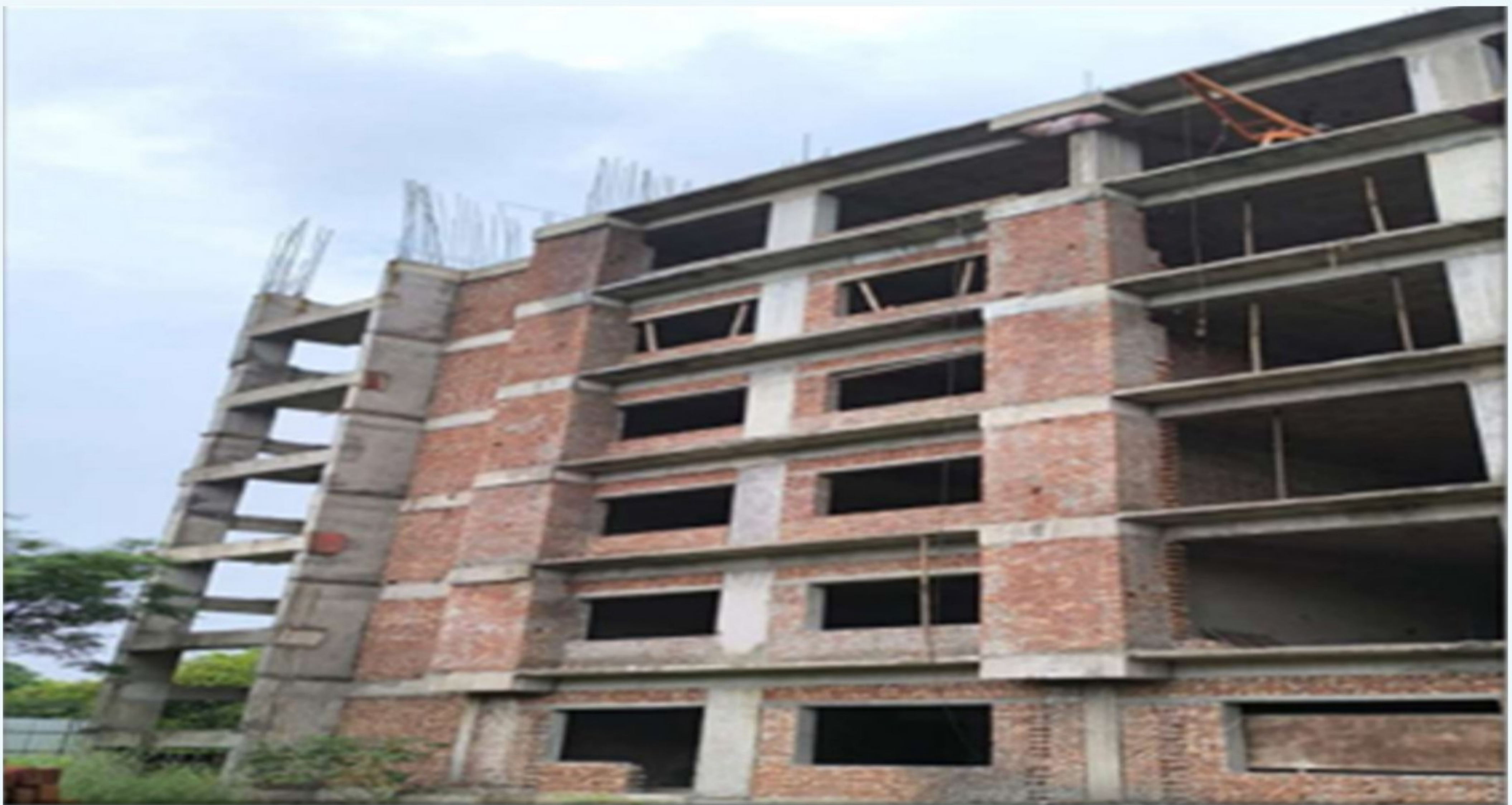
Project Construction, Jamiya Milia Islamia University – New Delhi
